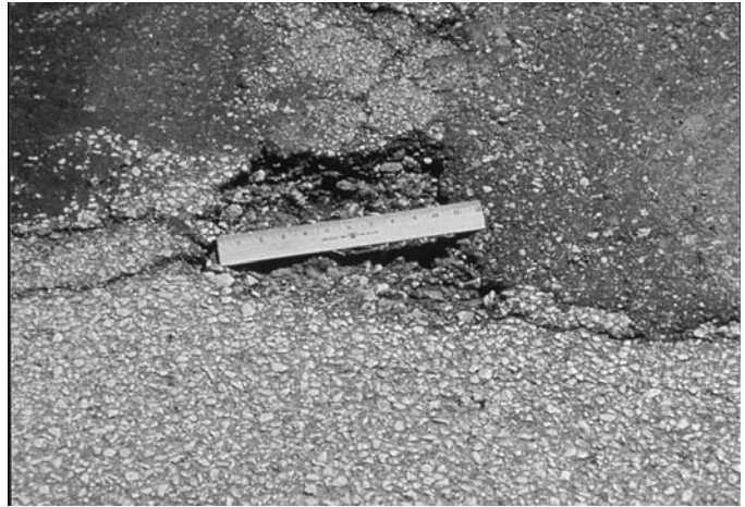
FIG. X1.35 Low-Severity Pothole
