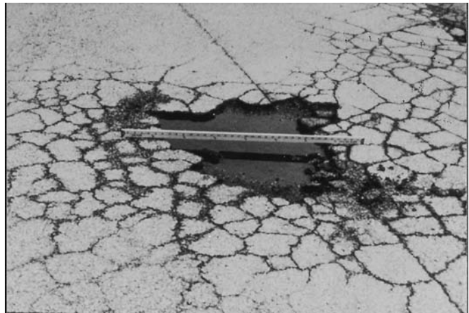
FIG. X1.37 High-Severity Pothole
