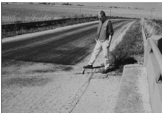
FIG. X1.44 Low-Severity Shoving
