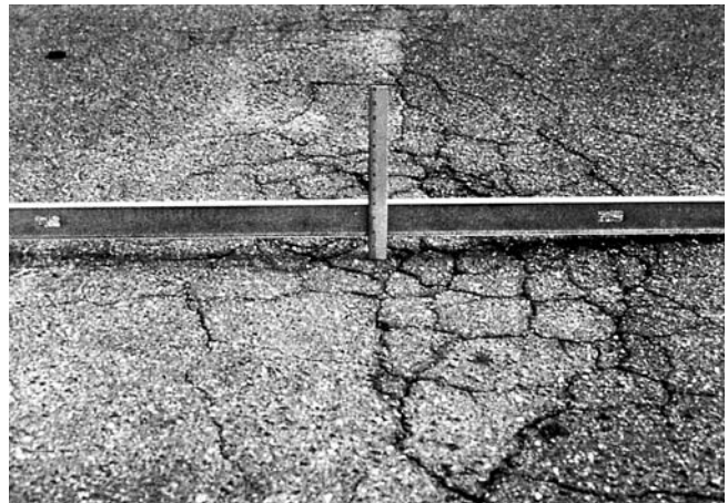
FIG. X1.18 High-Severity Depression
