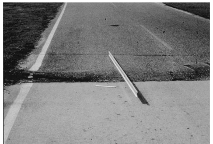
FIG. X1.46 High-Severity Shoving
