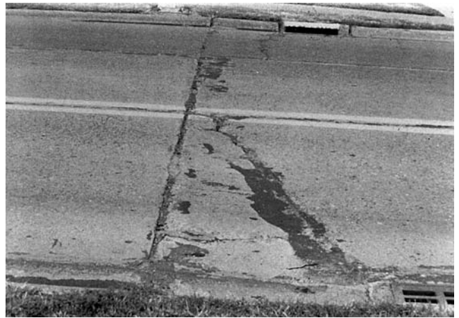
FIG. X2.36 Medium-Severity Punchout
