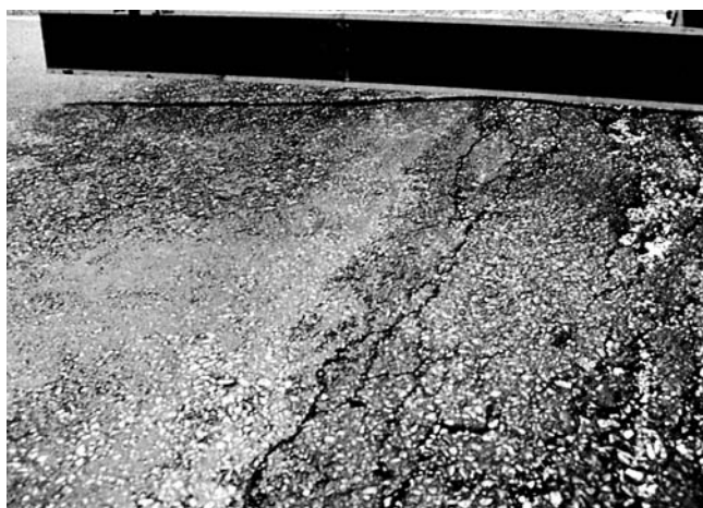
FIG. X1.12 High-Severity Bumps and Sags
