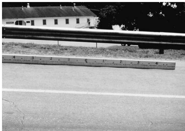
FIG. X1.13 Low-Severity Corrugation
