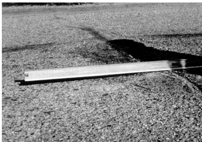
FIG. X1.10 Low-Severity Bumps and Sags
