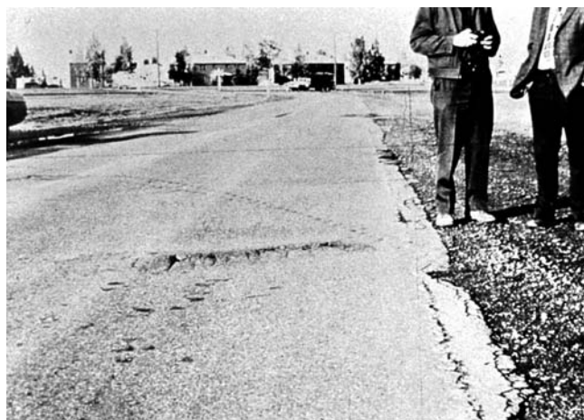
FIG. X1.11 Medium-Severity Bumps and Sags
