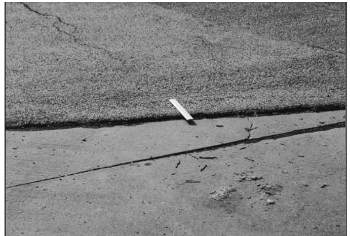
FIG. X1.45 Medium-Severity Shoving
