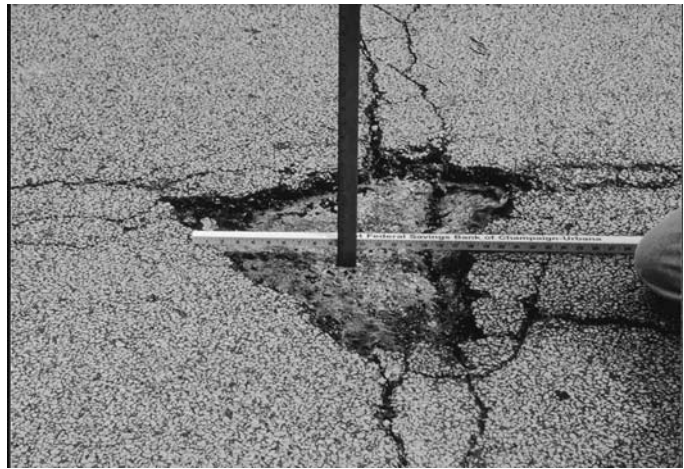
FIG. X1.36 Medium-Severity Pothole
