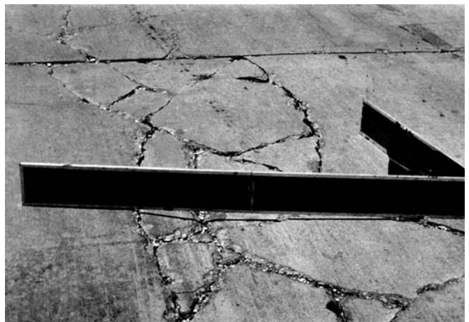
FIG. X2.37 High-Severity Punchout
