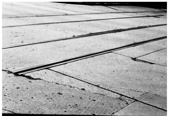
FIG. X2.38 Low-Severity Railroad Crossing
