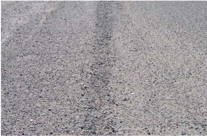
FIG. X1.52 High-Severity Raveling
