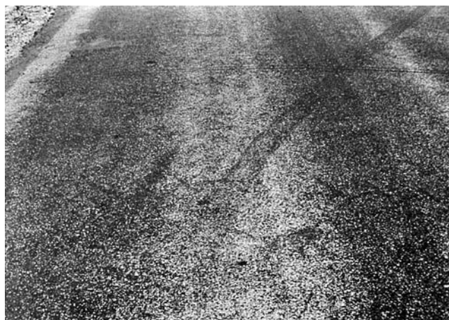
FIG. X1.4 Low-Severity Bleeding
