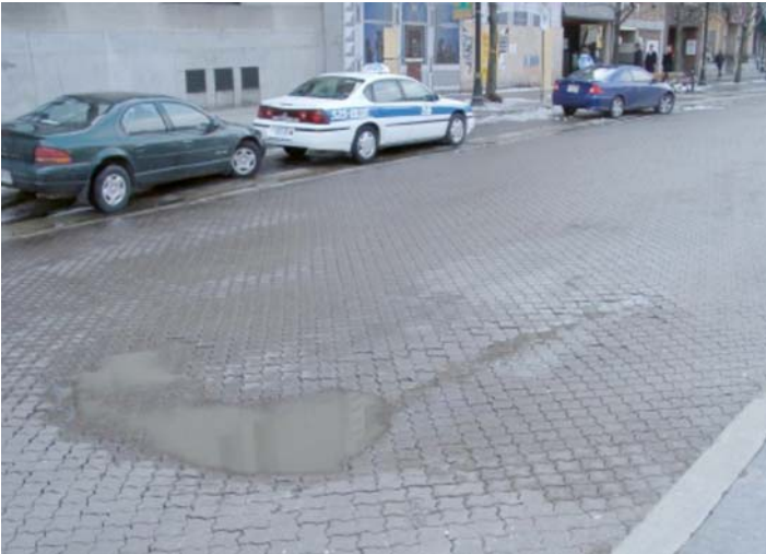
FIG. X1.6 High Severity Depression
